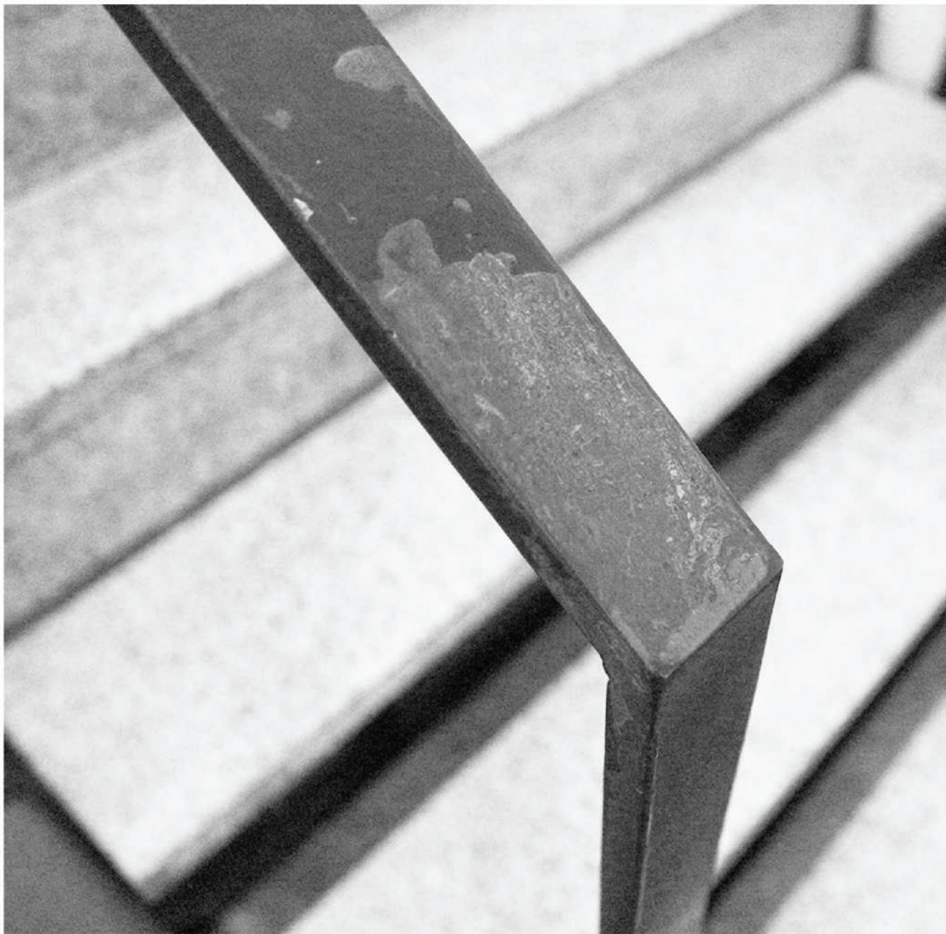
PICTURE 13. ADDITION RAILING WITH "FAKE" OLD / UNFINISHED EFFECT SOURCE : WRITER
