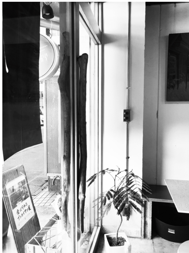
ENTRANCE SLIDING DOOR REUSED FROM EXISTING DOOR WITH THE ADDITION OF THE WOODEN HANDLE
